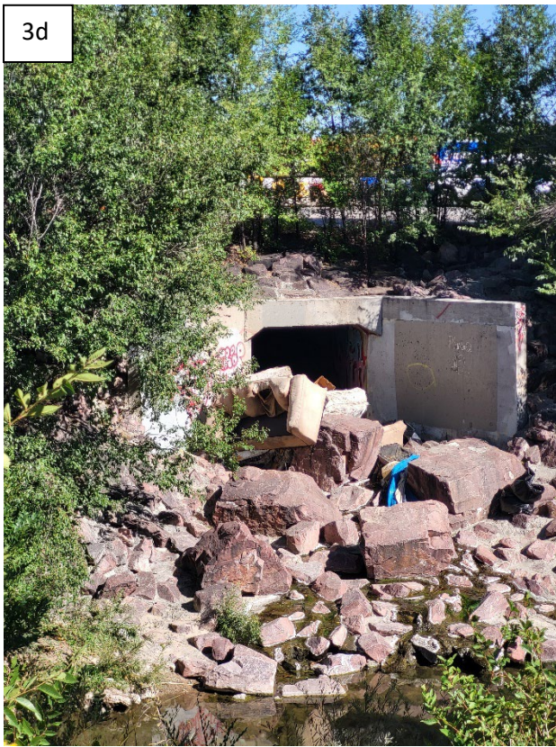
Figure 3d and f. Culvert and foot bridge crossing Creek both with solid waste accumulation.
