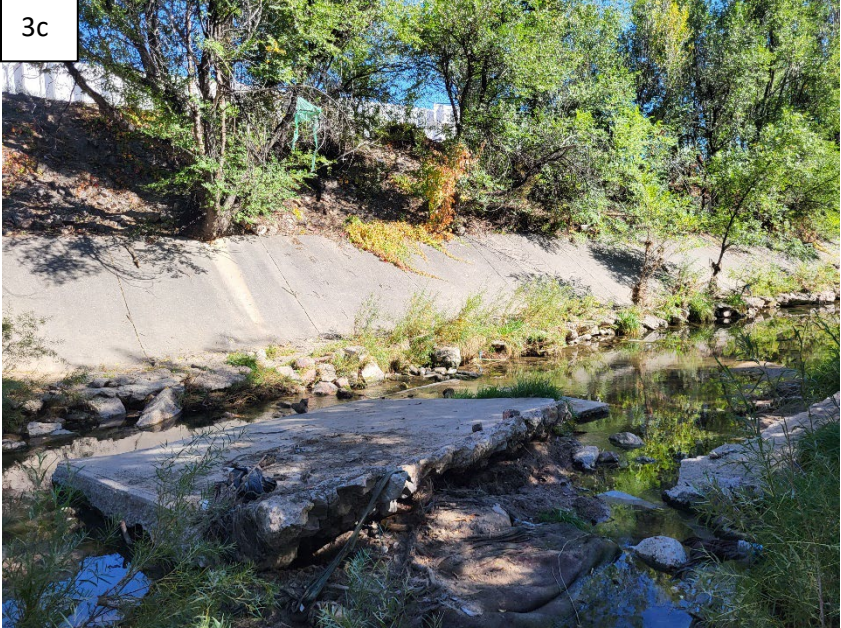
Figure 3a, b and c. Wier, concrete lined channelized section with concrete slab in river
